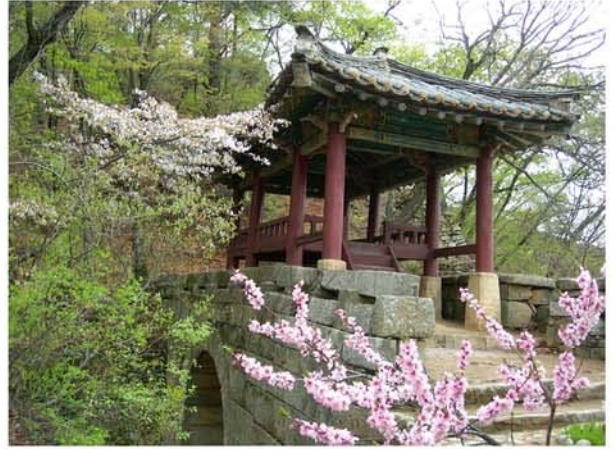
The north gate of the Taehungsan Fort.
